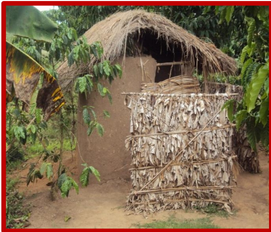
A pit latrine fitted with a shield wall.
